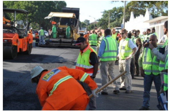
SAT members inspect WMA paving on a road in Greyville, Durban
