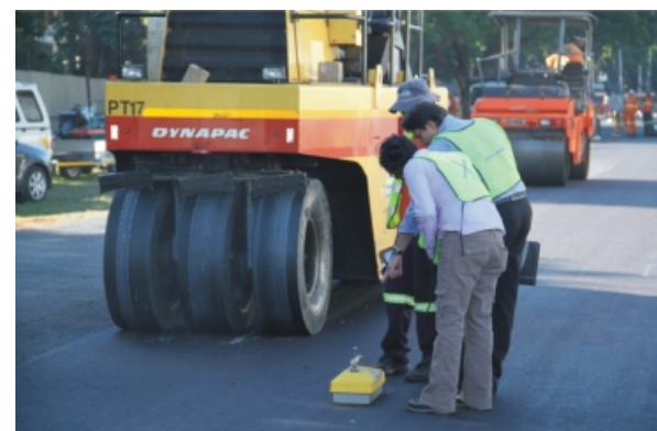
SAT WMA workshop delegates inspecting compaction of warm mix, Greyville, Durban
