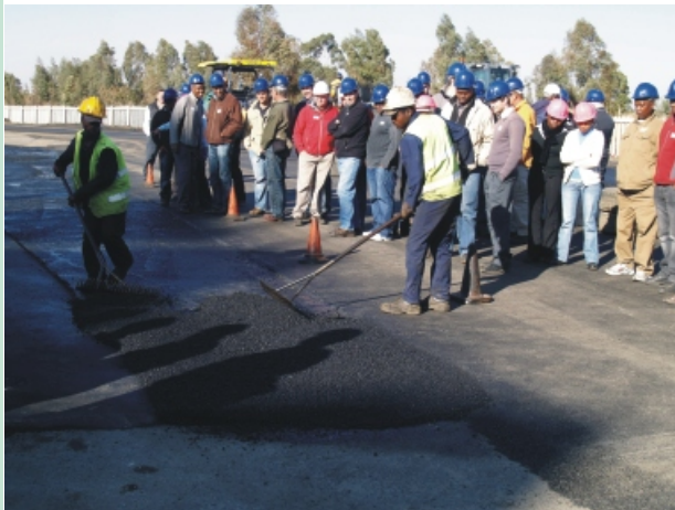
SAT delegates view hand placing of WMA
