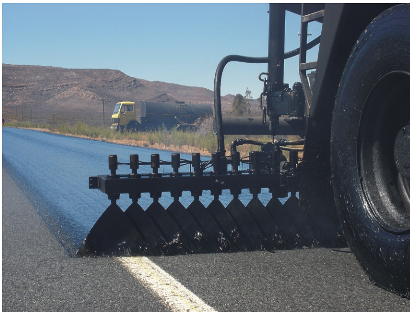
Bitumen emulsion may be sprayed at an accurately controlled rate onto a road surface before the application of gravel to improve surface condition and skid resistance.
