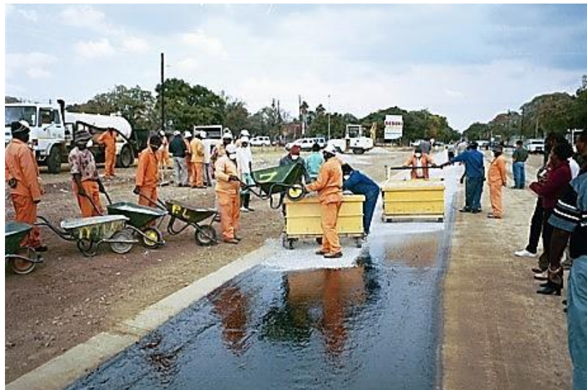
Photo 2: Application of stone aggregate with walk-behind spreaders
