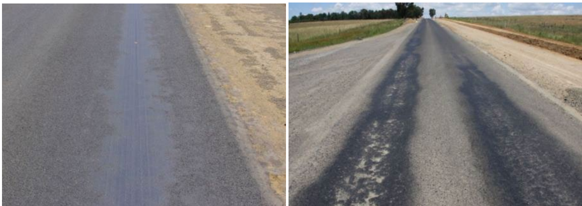
Figure 23 Open 20 mm structure allows 7 mm aggregate to force binder upwards
