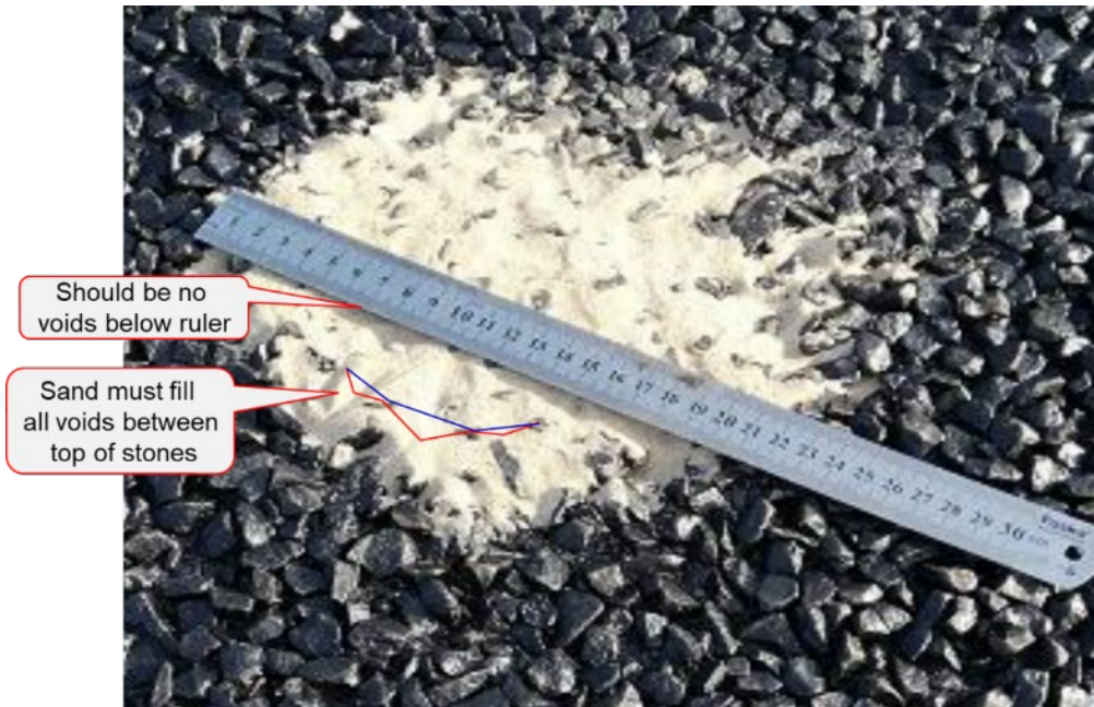
Figure 5 Sand not filling voids between stones
