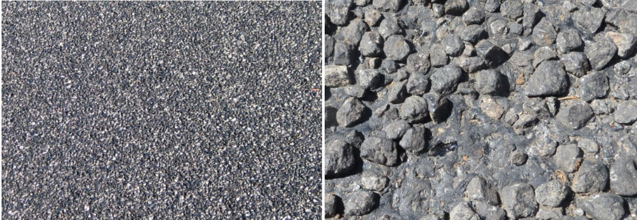
Figure 18 Result of volumetric design after construction and stripping within a week
