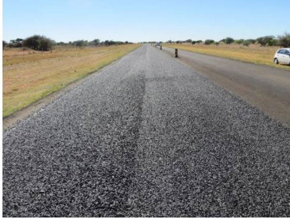
Figure 25 Difference in aggregate orientation with only PTR rolling versus PTR and steel wheel
