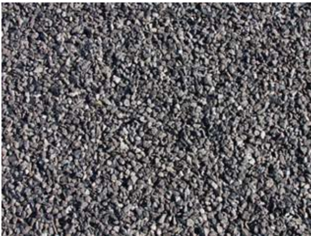
Figure 19 7 mm seal before cover spray of diluted 60% Anionic emulsion (50/50) at 1.0 l/m 2
