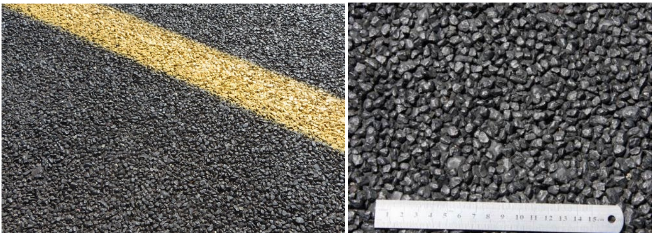
Figure 27 Full 20/10 double seal
