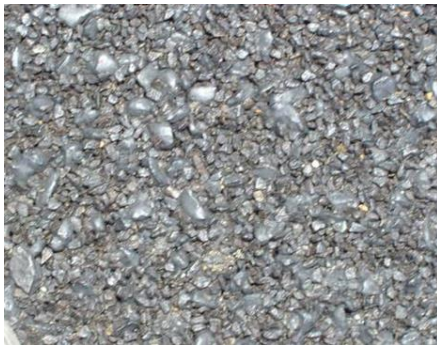
Figure D 23 Coarse 20/7 Double Seal
