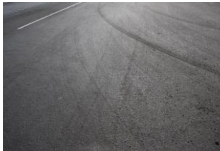
Figure D 14 Temporary 10 mm Cape Seal on Intersection
