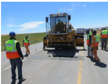
Figure F 30 Calibration of the Chip Spreader
