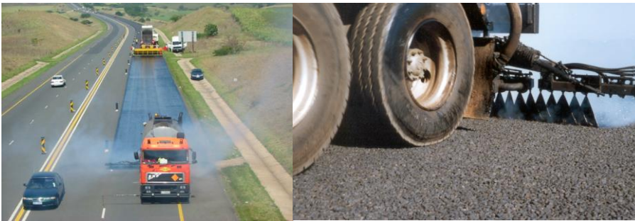
Figure F 1 Fixed Angled Flair Distributor
