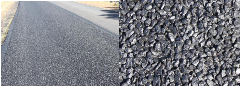
Figure F 32 Dense Matrix Obtained after Traffic Compaction/ Orientation
