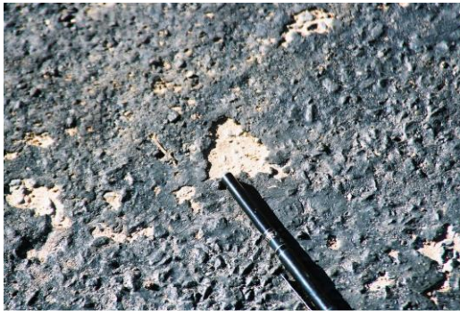
Figure F 39 Effect of Spraying Emulsion Before Cleaning
