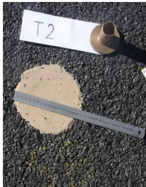
Figure H 14 Repair Using 7 mm Aggregate – Final Surface
