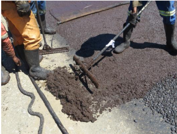
Figure F 44 Coarse Particles Segregating from the Slurry Mix
