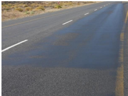
Figure E 51 Effect on Slurry Not Compensating for Bulking due to Moisture
