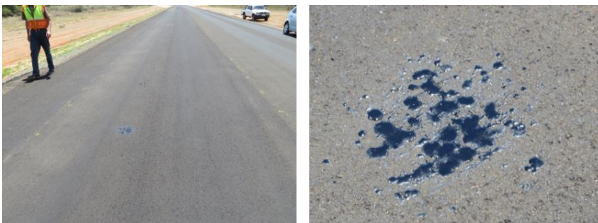
Figure H 5 Bleeding Cape Seal – 70/100 Pen Bitumen at 80°C Road Surface Temperature
