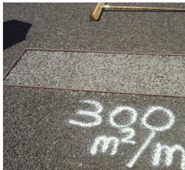
Figure F 28 Large Aggregate Visible after Spread of the Dry Layer
