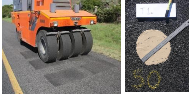
Figure H 11 Trials with different binder application rates (close-up of 1.1 l/m 2 )
