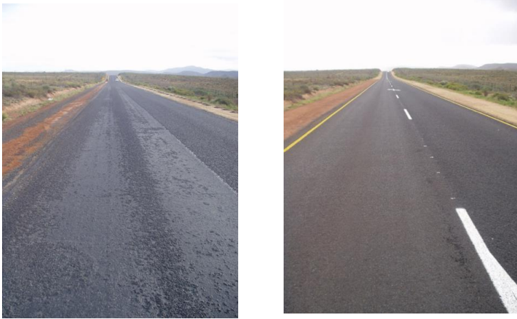
Figure H 24 Before and After repair
