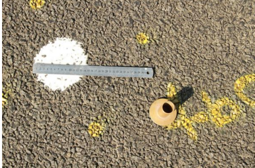
Figure H 18 N1/14 Section 4b – 20/10 Double Seal
