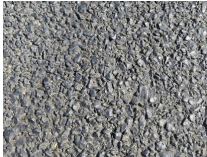
Figure H 7 Treated Stripped 14/7 Double Seal
