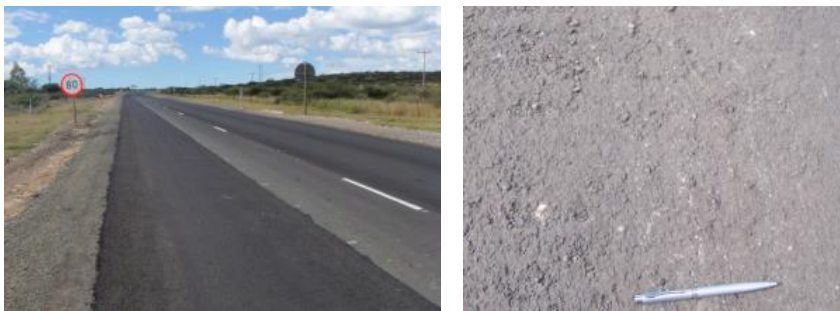
Figure D 15 Microsurfacing (8mm)
