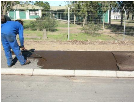
Figure D 26 Slurry Applied on Footway (Sidewalk)
