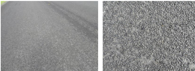
Figure H 9 Slight Losses but Uniform and Ideal for Small Aggregate Filling
