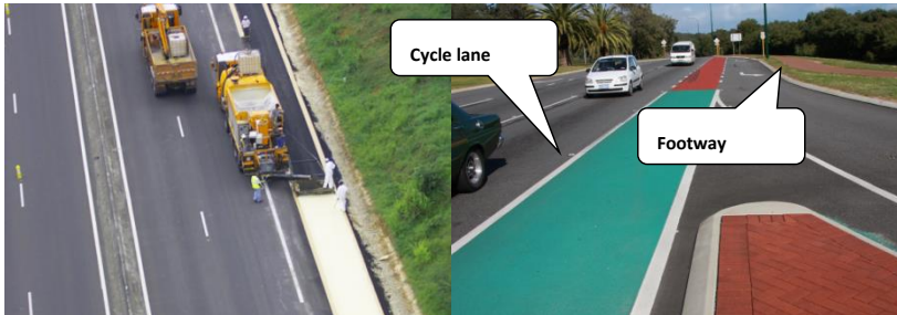
Figure D 27 Colored slurry on cycle lanes and footways (side walks)
