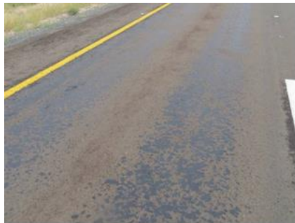
Figure E 47 Bleeding of a Cape Seal through a Ravelling Slurry
