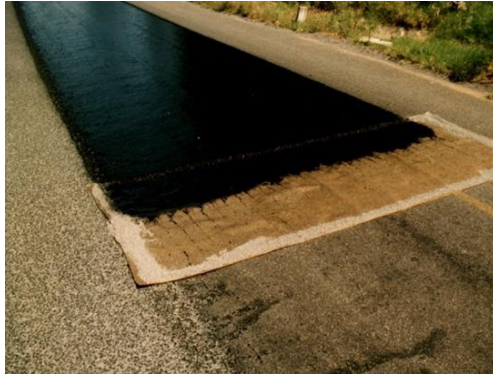
Figure F 21 Transverse Joint
