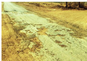
Figure C 19 Sensitivity of a Single Sand Seal at Intersections
