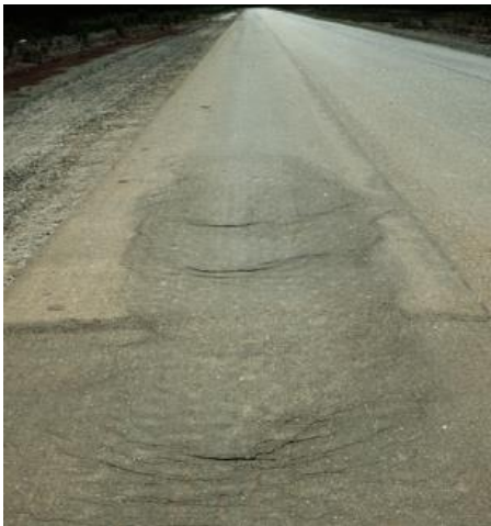
Figure D 7 Shoving of Slurry on a Smooth Substrate
