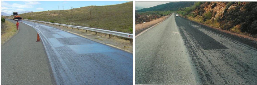
Figure C 40 Effect of Sealing on Different Existing Textures
