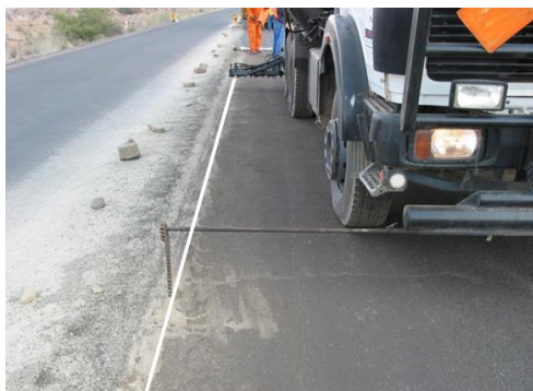
Figure F 18 Guide Marker on String Line
