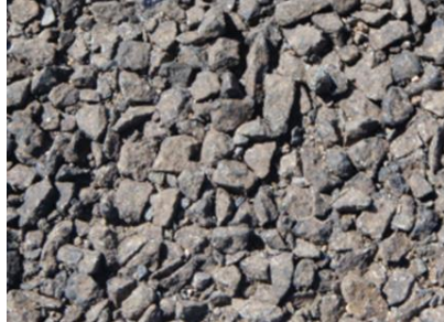
Figure D 11 Temporary 10 mm Single Seal without Emulsion Cover Spray
