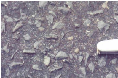
Figure E 14 Texture of a Cape Seal
