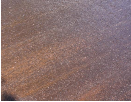
Figure F 37 Emulsion Forced to the Surface Due to Too Early Rolling
