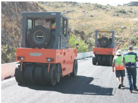
Figure F 3 Pneumatic Tyre Rollers
