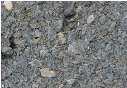
Figure C 24 Dry/Brittle Double Seal
