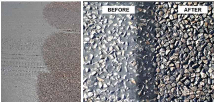
Figure H 28 Examples of the Effect of Hydro-Cutting
