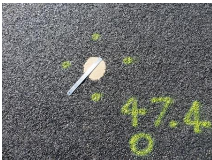
Figure D 24 Fine 20/7 Double Seal
