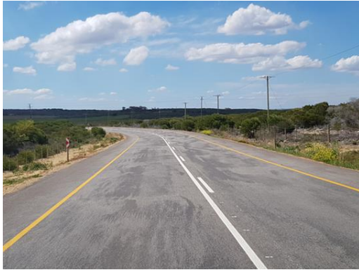
Figure F 45 Effect of Coarse Particle Segregation
