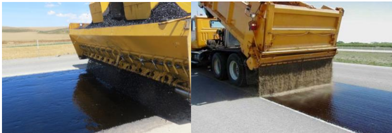
Figure F 2 Self-Propelled and Non-Self-Propelled Chip Spreader
