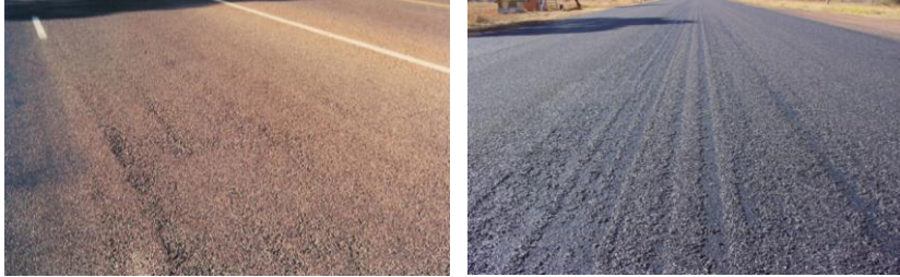
Figure C 41 Implication of Not Pre-treating a Variable Existing Surface
