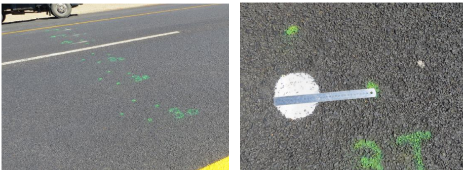
Figure H 17 Repaired 20/10 Double Seal
