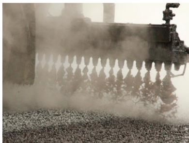
Figure C 35 Too High Viscosity Emulsion
