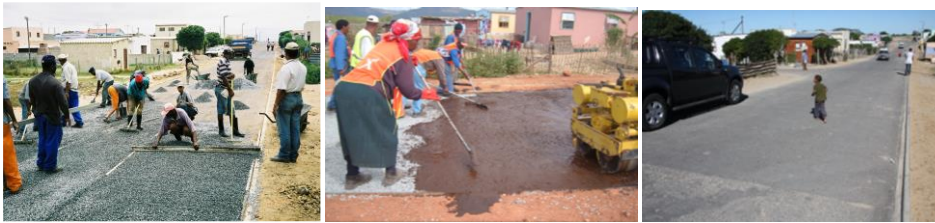
Figure D 18 Slurry Bound Macadam
