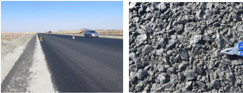
Figure H 16 Stripping of the 10mm Aggregate From a 20/10 Double Seal
