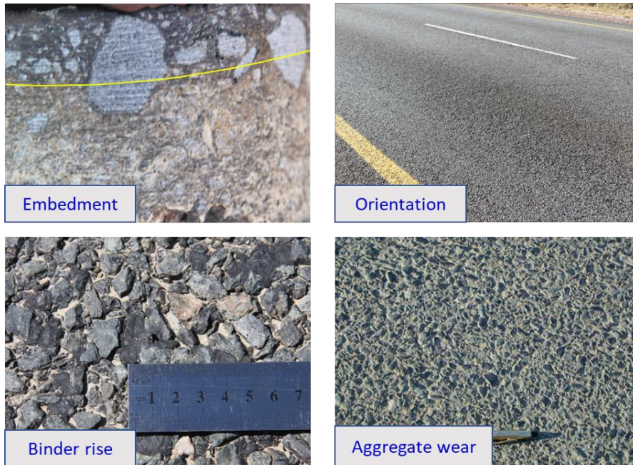
Figure C 45 Causes of Texture Loss
