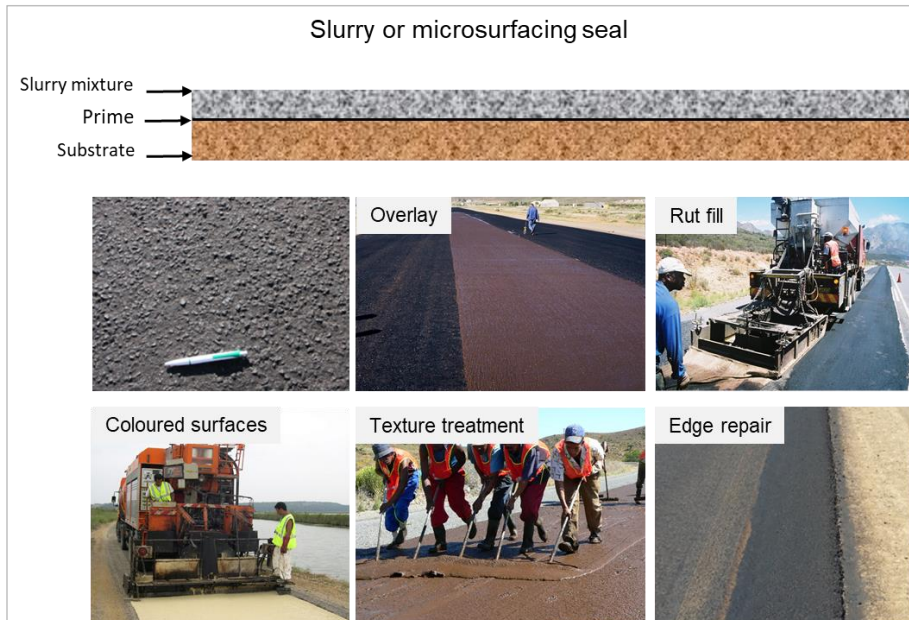
Figure A 20 Slurry and Microsurfacing Applications
