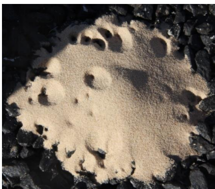
Figure H 13 Sand Trickle into Porous Surfacing
