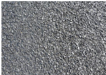
Figure H 6 Non-Stripped 14/7 Double Seal Texture
