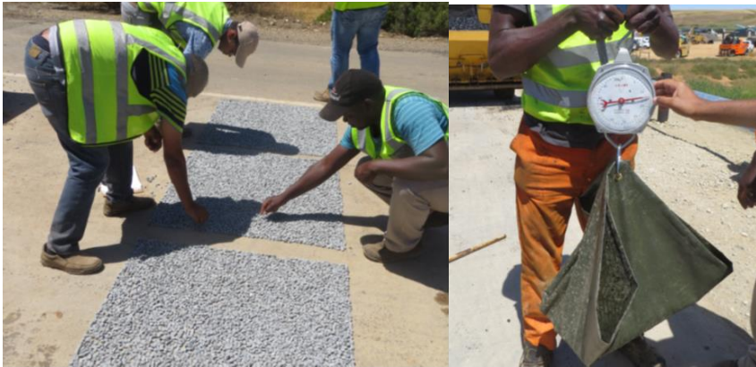
Figure F 29 Determining Appropriate Aggregate Spread Rate on Site
