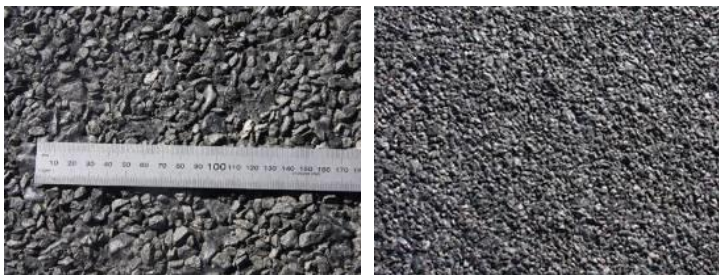
Figure H 12 Before and After (Slow Lane at 0.9 l/m 2 )
