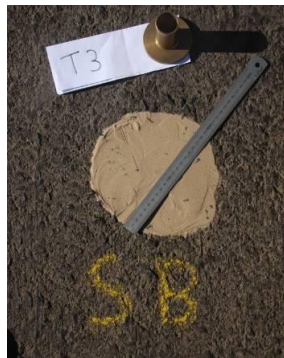
Figure H 15 Repair Using a Fine Slurry
