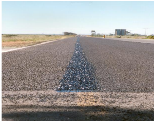
Figure F 24 Additional Joint Over Spray
