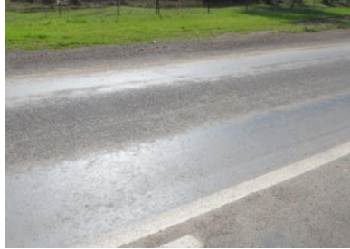
Figure E 13 High Variation in Macro Texture Depth
