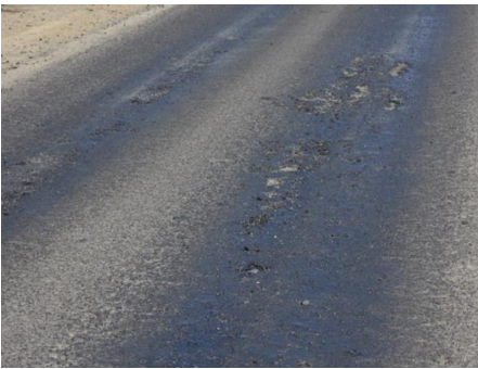
Figure D 9 Reseal Applied too soon after Rejuvenation Spray
