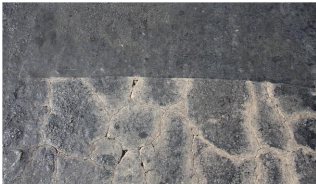
Figure C 42 Ability of a Bitumen Impregnated Geotextile to Retard Crack Reflection
