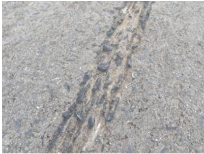
Figure D 21 Loss of Low Binder Content Slurry
