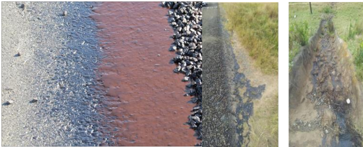
Figure C 30 Run-Off of Low Viscosity Emulsions
