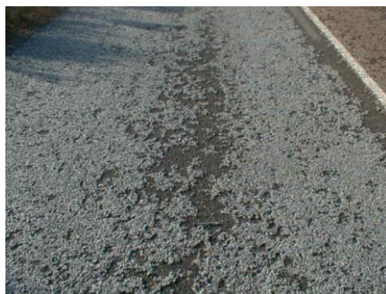
Figure E 24 Stripping of Quarzitic Aggregate
