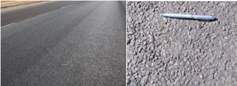
Figure D 12 Single 10 mm Seal with Emulsion Cover Spray (N1/14 after 1 year)
