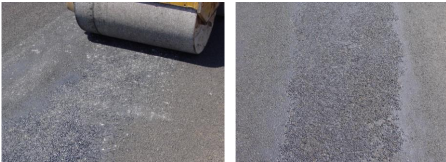
Figure H 26 Rolling-in of Aggregate and Finished Treatment
