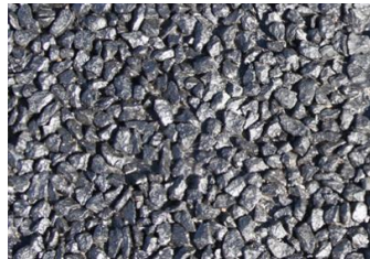
Figure E 29 Dense Shoulder-to-Shoulder Matrix after Construction and Traffic Compaction
