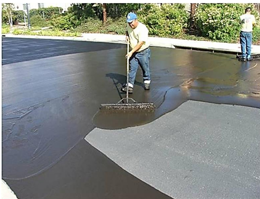
Photo 3: Application of slurry with squeegees
