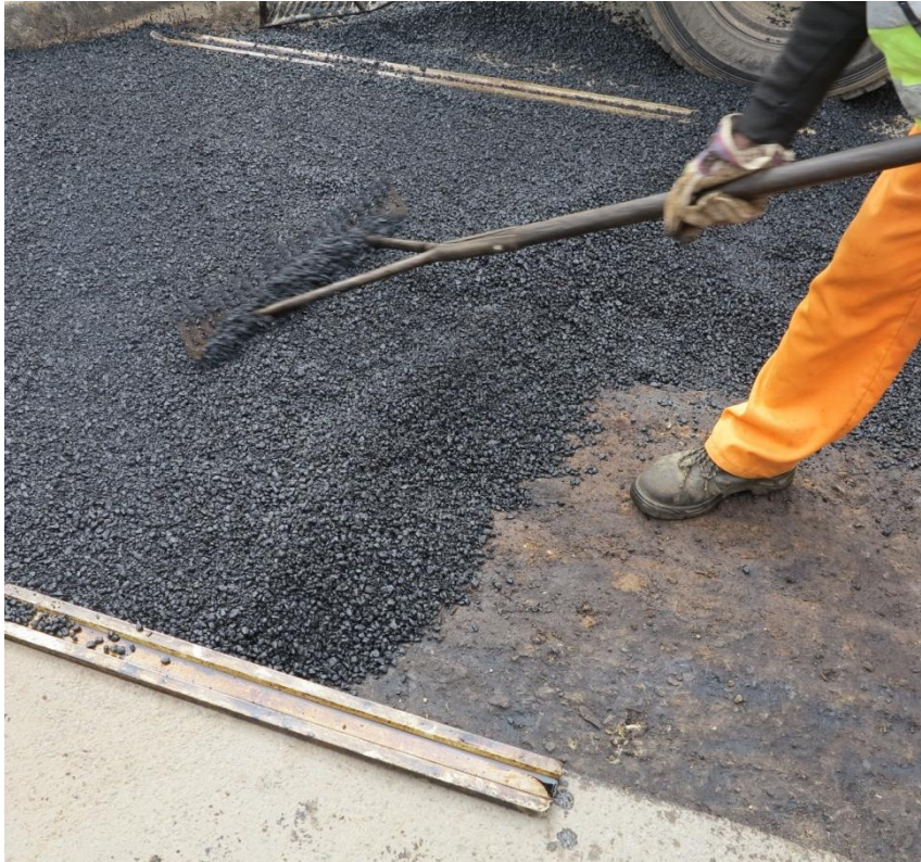
Photo 7: Hand-spreading of asphalt between channels
