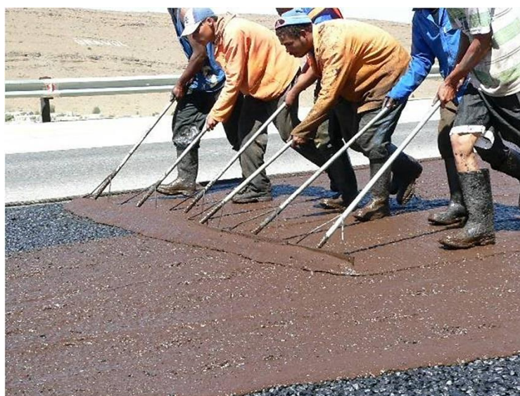
Photo 4: Applying slurry as a seal filler
