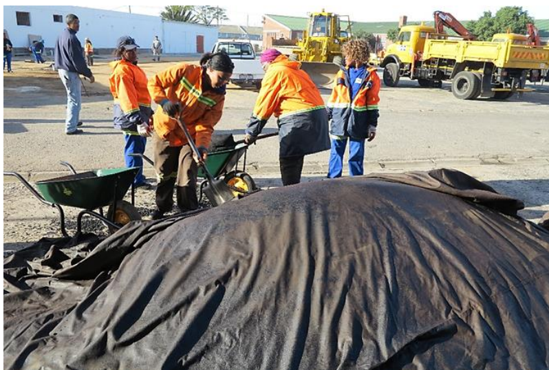
Photo 6: Hot asphalt covered with tarpaulins
