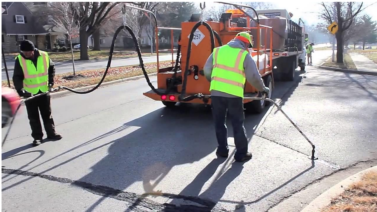
Photo 10: Applying sealant to prepared crack
