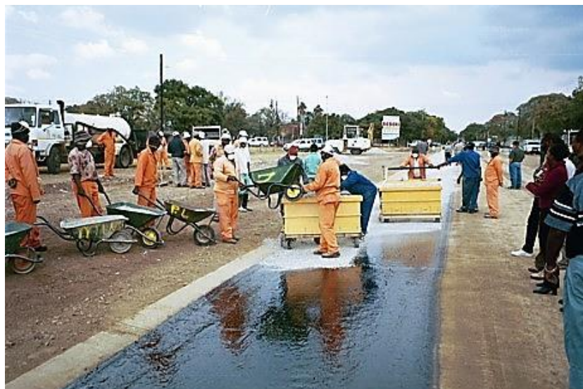
Photo 2: Application of stone aggregate with walk-behind spreaders
