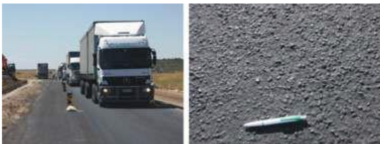
Photograph 5: Temporary 9,5 mm Cape seal after one year
