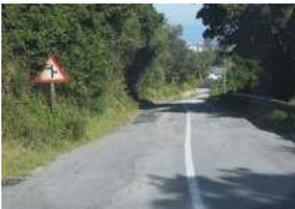
30 mm asphalt on steep grades >20 years
