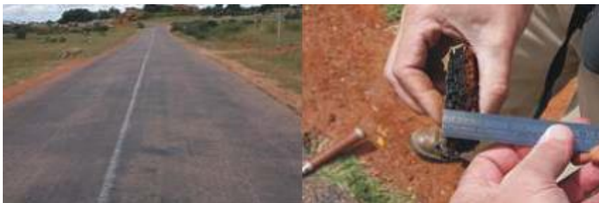
Thick single Otta seal (>15 mm) with high fines content
