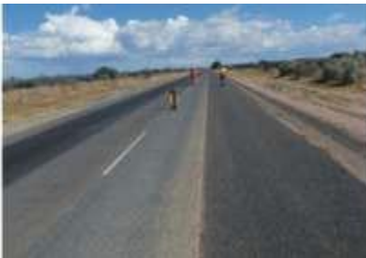
Photograph 2: Temporary 9,5 mm single seal without emulsion cover spray
