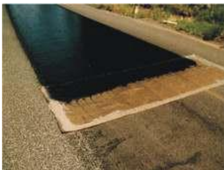
Photograph 16: Use of joint paper at transverse joint
