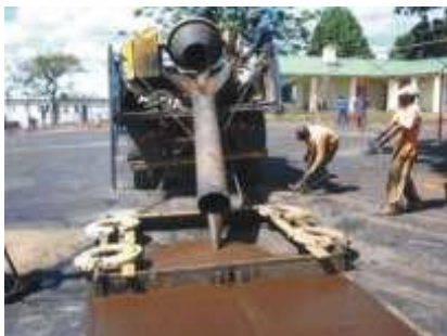
Photograph 8: Small scale slurry operation
