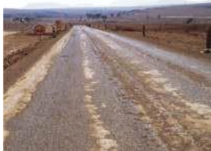
Photograph 1: Single 13,2 mm seal without cover spray
