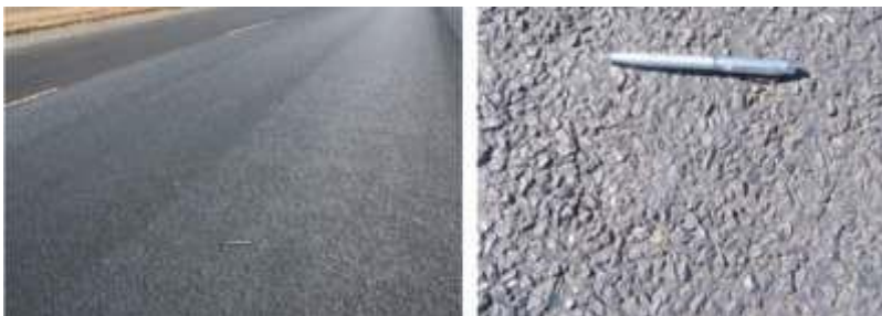
Photograph 3: Single 9,5 mm seal with emulsion cover spray (N1/14 after 1 year)
