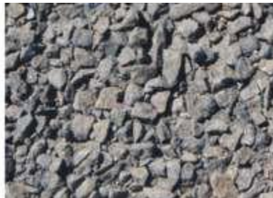
Photograph 2: Temporary 9,5 mm single seal without emulsion cover spray
