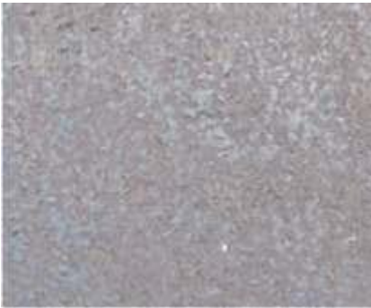
Photograph 7: 9,5 mm single seal with natural fine sand blinding
