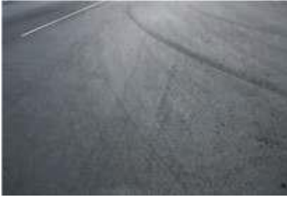
Photograph 6: Temporary 9,5 mm Cape seal on an intersection
