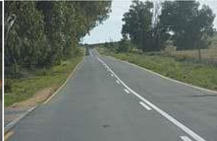
12 mm UTA resurfacing low speed rural road
