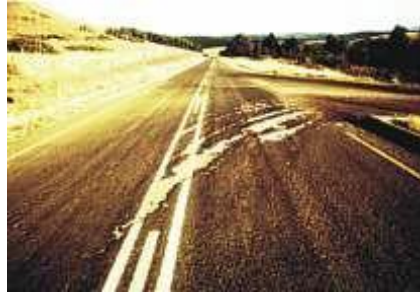
Aggregate loss on single seal due to turning actions
