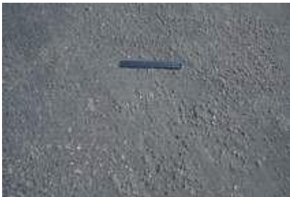
9,5 mm Cape seal on intersection (after 9 years)
