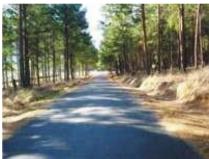
Photograph 9: Slurry surfacing on forestry road
