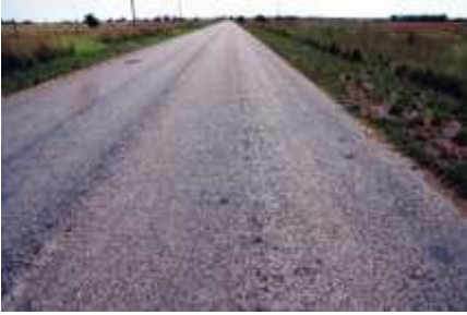
Graded aggregate seal (minus 13,2 mm with low fines content) after 8 years
