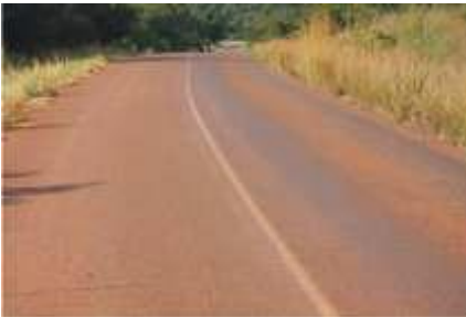
Dust palliative resealed after 3 years with 9,5 mm single seal (20 years later)
