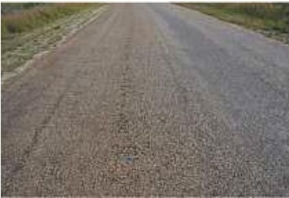
13,2 mm single seal after 11 years on properly constructed base
