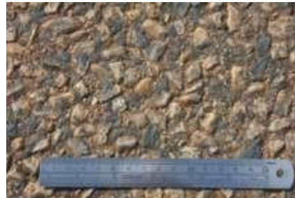
No defects apart from brittle binder
