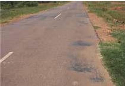
13,2 mm plus high fines sand seal after 6 years. Labour intensive construction
