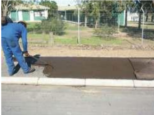
Photograph 10: Slurry applied on footway (side walk)
