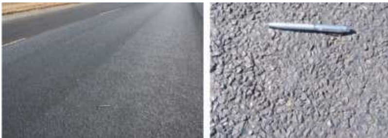
Photograph 4: Microsurfacing (8 mm)
