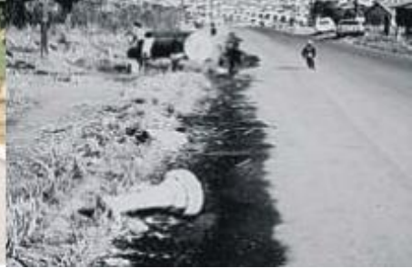
40 mm asphalt effective in preventing damage due to building rubble
