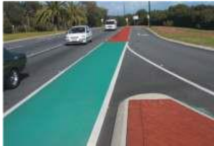
Photograph 12: Cycle lane and footway coloured surfaces
