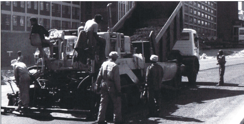
Paving of asphalt.
