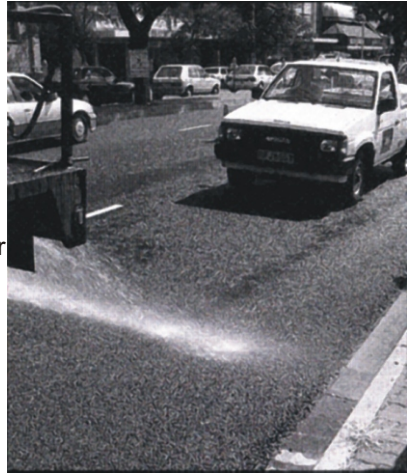
Porosity test conducted on a porous asphalt: water immediately penetrates into the layer.
