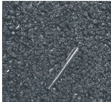
Texture of well-constructed porous asphalt.
