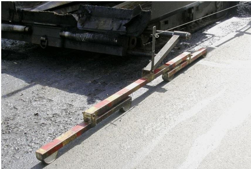
Figure 27: Mechanical Sensor on Articulated Averaging Beam
