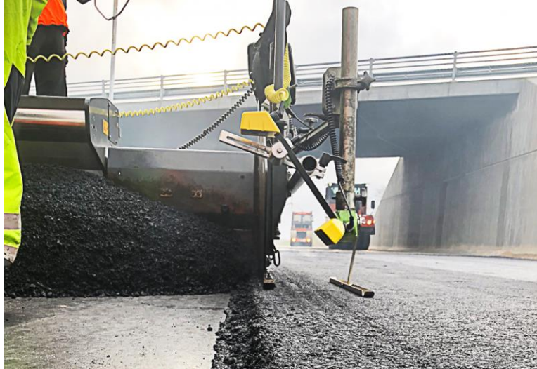
Figure 30: Joint Matching Shoe (contact type)
