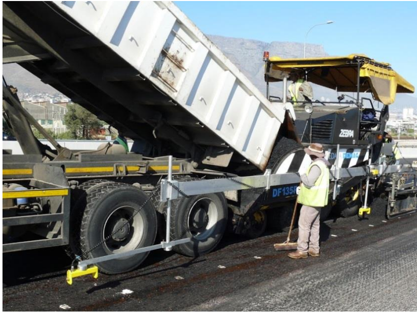
Figure 28: Two-Level Articulated Averaging Beam
