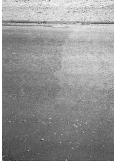
Crack sealing with slurry
