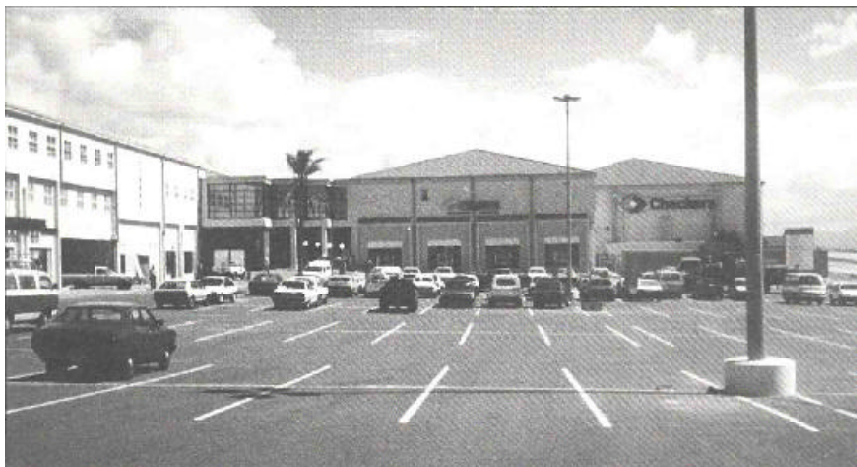
Wearing course alternative to large shopping complex in Port Elizabeth
