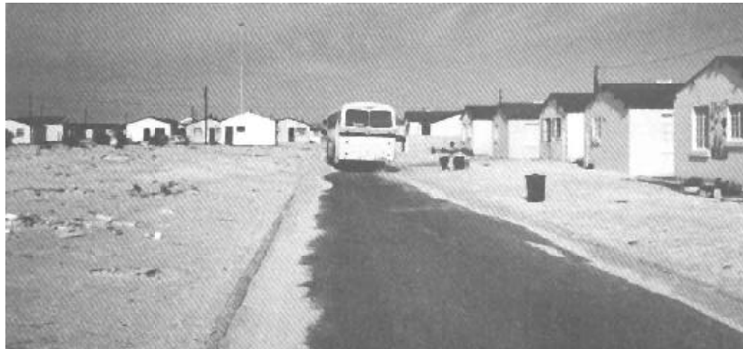
Access to residential areas for lower income group housing developments in Khayelitsha, Cape
