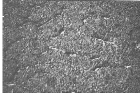
Fatigue cracking in sand asphalt
