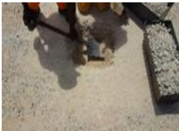
Figures A10 (a) and (b): Extracting all Loose Material and Transferring to Containers
