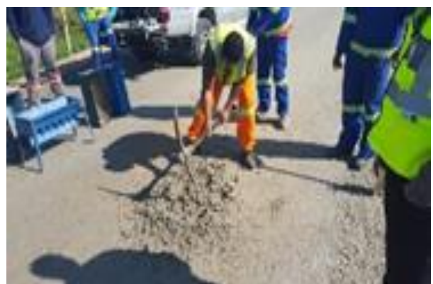
Figure A9: Using a Pick to Loosen the Material and Dig through the Entire Layer
