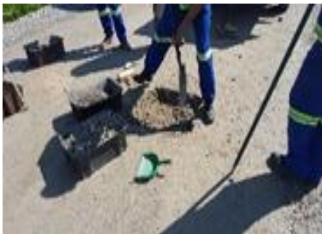
Figures A10 (a) and (b): Extracting all Loose Material and Transferring to Containers
