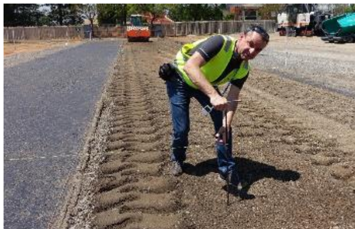
Figure 6.6 Checking the Cut Depth by Dipping
