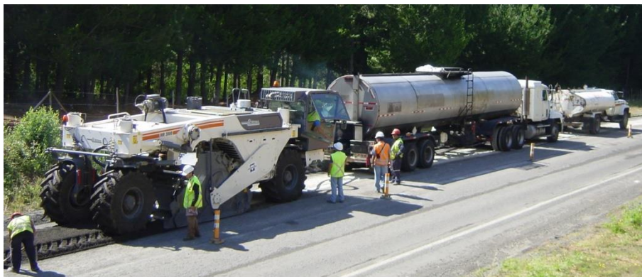
Figure 6.5 Typical Recycling Train for Bitumen Stabilisation
