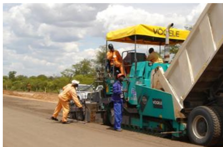
Figure 6.10 Paving the Second Half-Width
