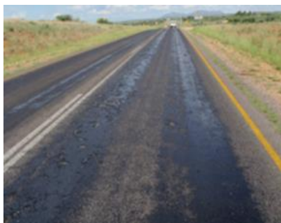
Figure H 4 Bleeding as a Result of Volatile Evaporation from Rejuvenation Treatment
