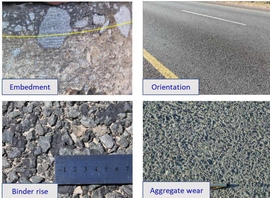
Figure C 45 Causes of Texture Loss
