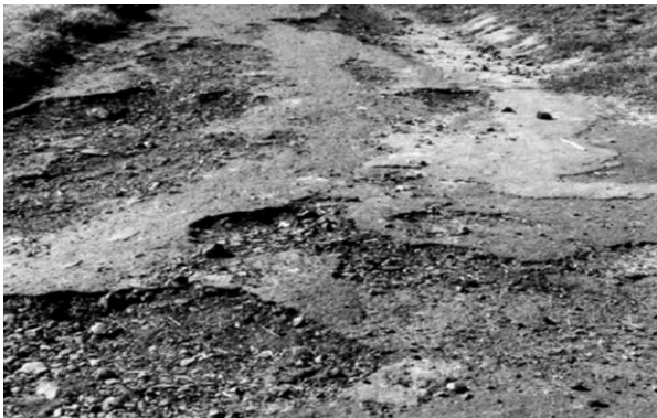
Figure C 17 Erosion of a Double Seal in a Wet Hilly Urban Environment
