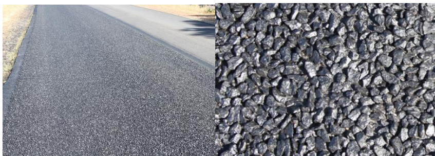
Figure F 32 Dense Matrix Obtained after Traffic Compaction/ Orientation
