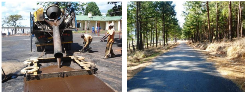
Figure D 25 Small Scale Slurry Operation and Completed Product
