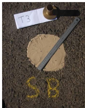
Figure H 15 Repair Using a Fine Slurry
