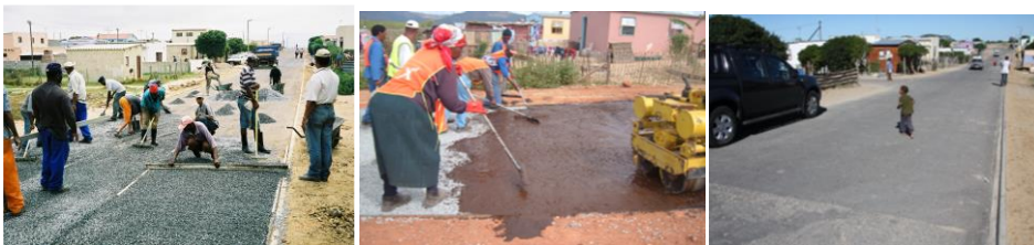
Figure D 18 Slurry Bound Macadam
