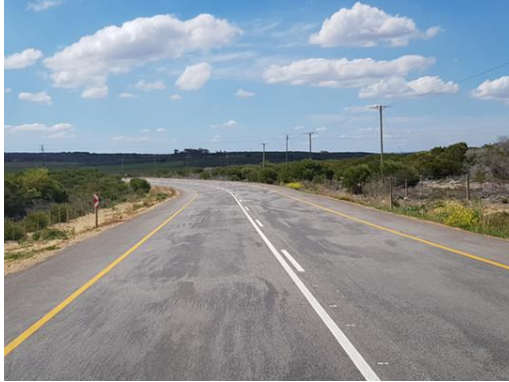
Figure F 45 Effect of Coarse Particle Segregation
