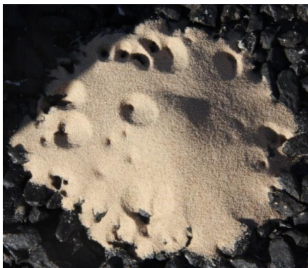
Figure H 13 Sand Trickle into Porous Surfacing
