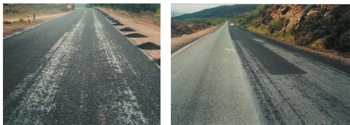
Figure H 23 Severe and Complete Loss of Aggregate
