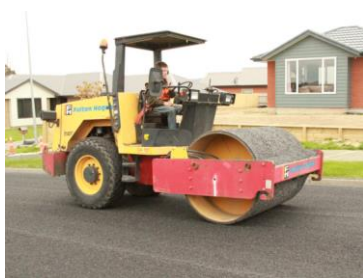
Figure F 4 Rubber Padded Steel Wheel Roller
