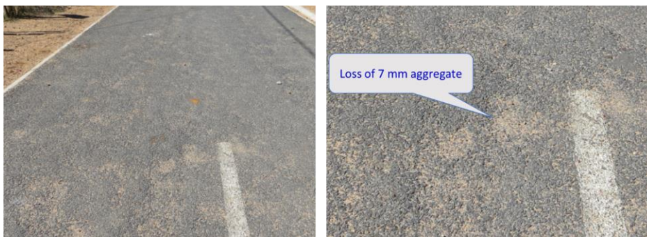
Figure C 13 Loss of 7 mm Aggregate on a S2(14/7) Double Seal due to Poor Compaction
