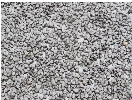
Figure F 31 Open Matrix after Rolling
