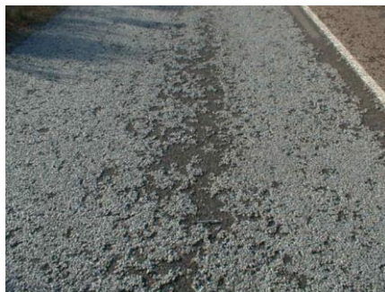
Figure E 24 Stripping of Quarzitic Aggregate
