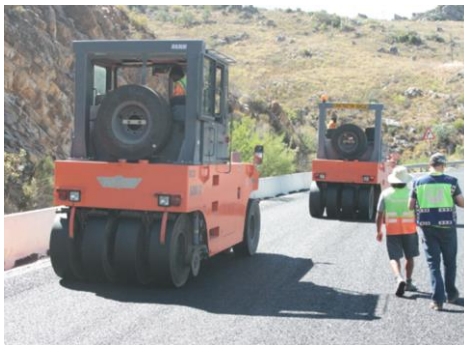
Figure F 3 Pneumatic Tyre Rollers
