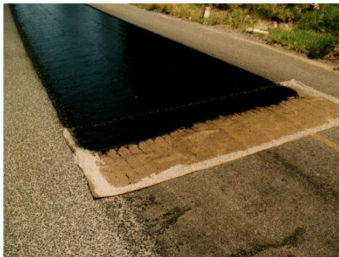
Figure F 21 Transverse Joint
