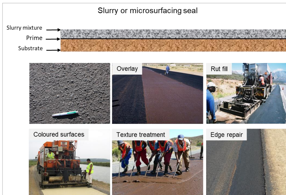
Figure A 20 Slurry and Microsurfacing Applications
