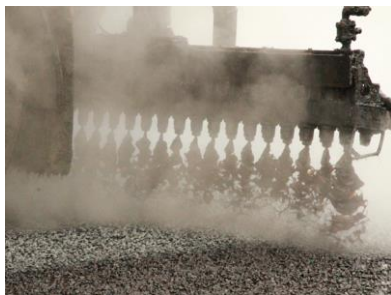
Figure C 35 Too High Viscosity Emulsion
