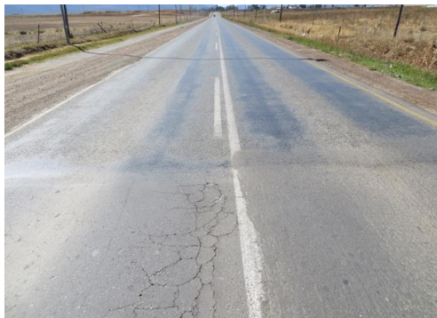
Figure C 15 S2(20/7/7) Geotextile Seal with S-E1 Compared with 40mm AC after 10 Years
