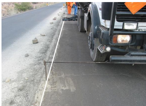
Figure F 18 Guide Marker on String Line
