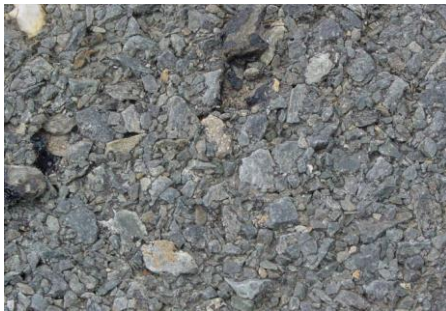
Figure C 24 Dry/Brittle Double Seal
