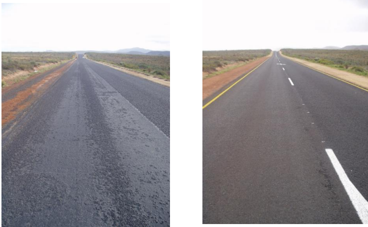
Figure H 24 Before and After repair
