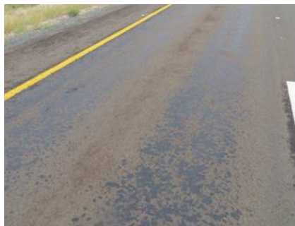
Figure E 47 Bleeding of a Cape Seal through a Ravelling Slurry
