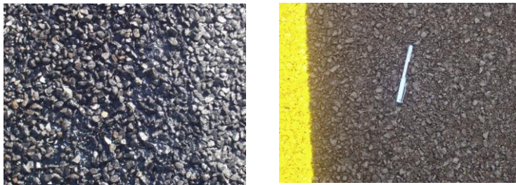
Figure H 25 After Application of Coarse Aggregate and the Final Repaired Surface
