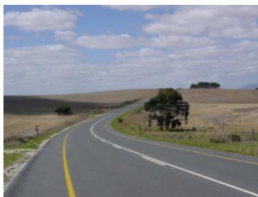
Figure D 6 Pre-coated Grit Seal with MC3000 as Binder
