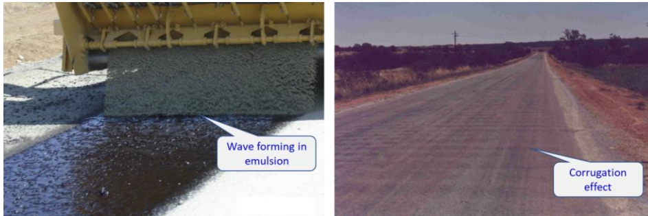
Figure F 47 Effect of Spreading Sand in Wet Emulsion
