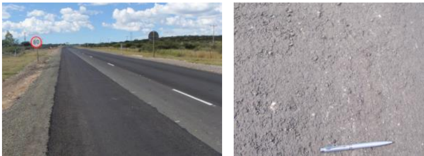
Figure D 15 Microsurfacing (8mm)
