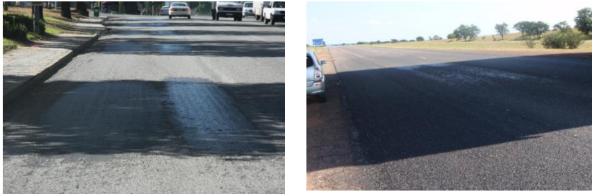
Figure H 2 Stripping Occurring Only in Shady Areas
