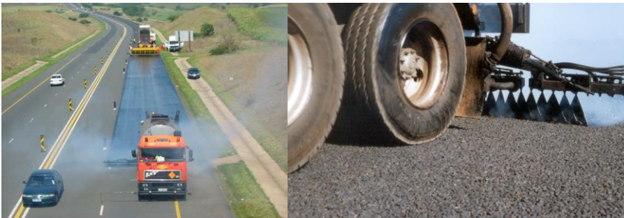
Figure F 1 Fixed Angled Flair Distributor
