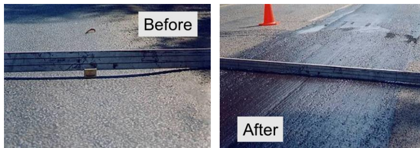
Figure F 35 Slurry Thickness to Compensate for Compaction
