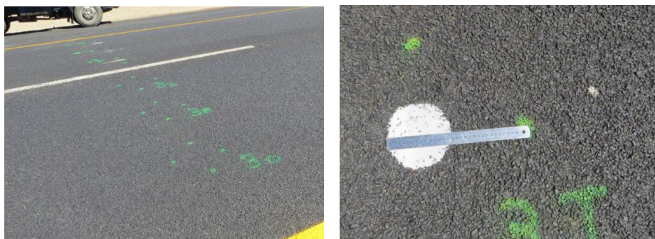
Figure H 17 Repaired 20/10 Double Seal
