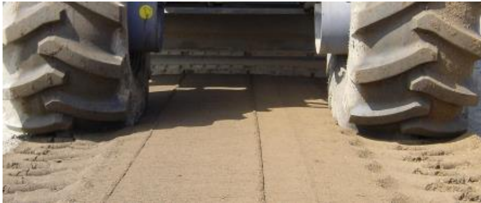
Figure 6.7 Mixed Material Exiting behind the Recycler
