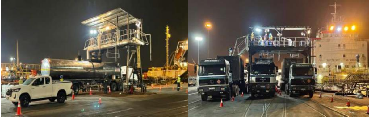
Figure 2 – Ship to shore discharge using a mobile gantry discharge system positioned on the quay alongside the vessel. The mobile unit usually includes a manifold with multiple loading arms that allows more than one road tanker to be loaded simultaneously. (Images courtesy of Colas South Africa)
